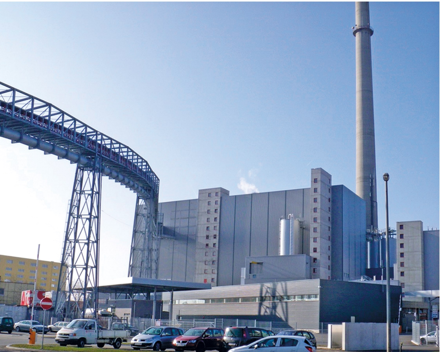
RHKW Linz – belt conveyor and incineration air pipe connecting the “Material Recovery Facility” to the boiler house (© Linz Strom GmbH)
