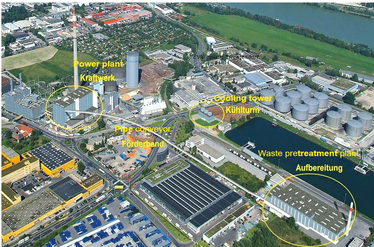
RHKW Linz – site integration of residue-based heat-and-power plant including cooling tower and pipe conveyor from mechanical waste treatment center "Material Recovery Facility" (© Linz Strom GmbH)
