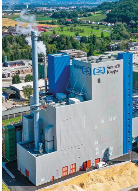
SKN Nettingsdorf Black Liquor Boiler (2020) 177 MW
