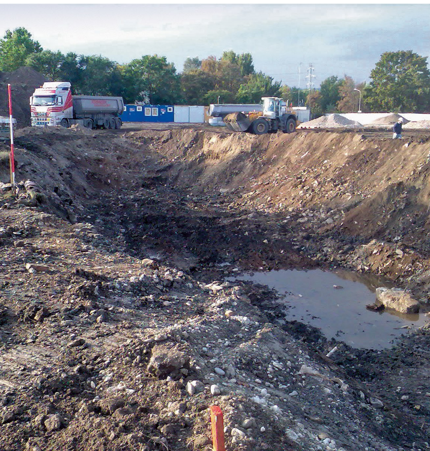
Excavation of contaminated material (© UVP GmbH)
