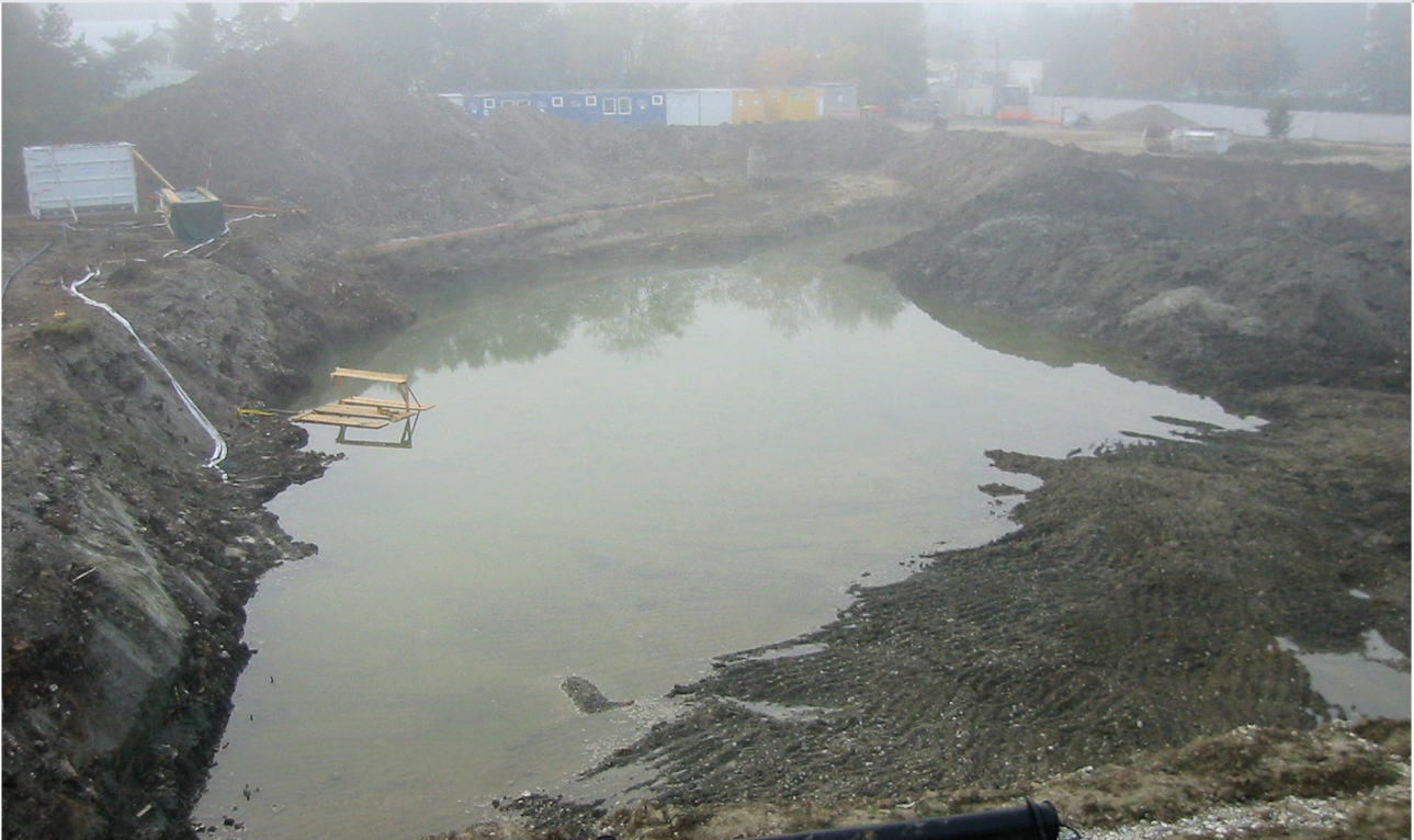
Remediation measures in groundwater fluctuation zone (© UVP GmbH)
